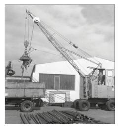
1962: Rope-driven S833 with elevated operator cab
