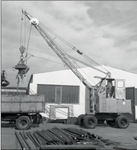
1962: rope-driven S833 with elevated operator cab
