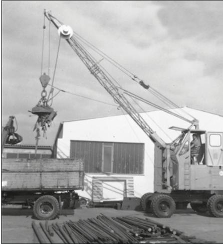
1962: Rope-driven S833 with elevated operator cab
